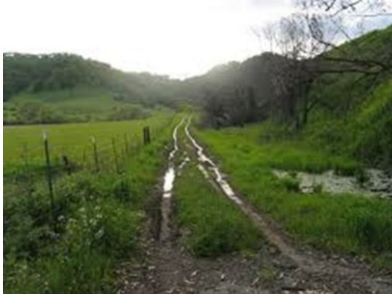
Figure 6. Rutting. Visual evidence of the collapse of soil. Notice the damming of water resulting from non-penetration.
